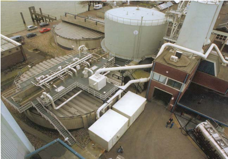
Figure 12 Reactor left, methane storage background
