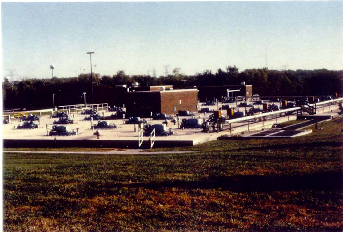
Original UNOX R nitrification reactors
